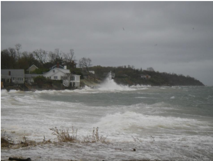
Figure 7. 21815 Soundview Avenue. Storm waves strike vertical bulkheads with explosive force jetting up massive and repetitive sea sprays that can be over 20 ft. in height and capable of attacking and eroding bluffs above bulkheads. 10/29/2012
